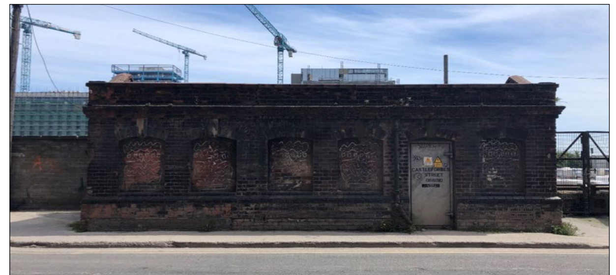
Figure 4.10: Detached single storey electricity substations external to the site on Castleforbes Road. Source: TPA, May 2020.
