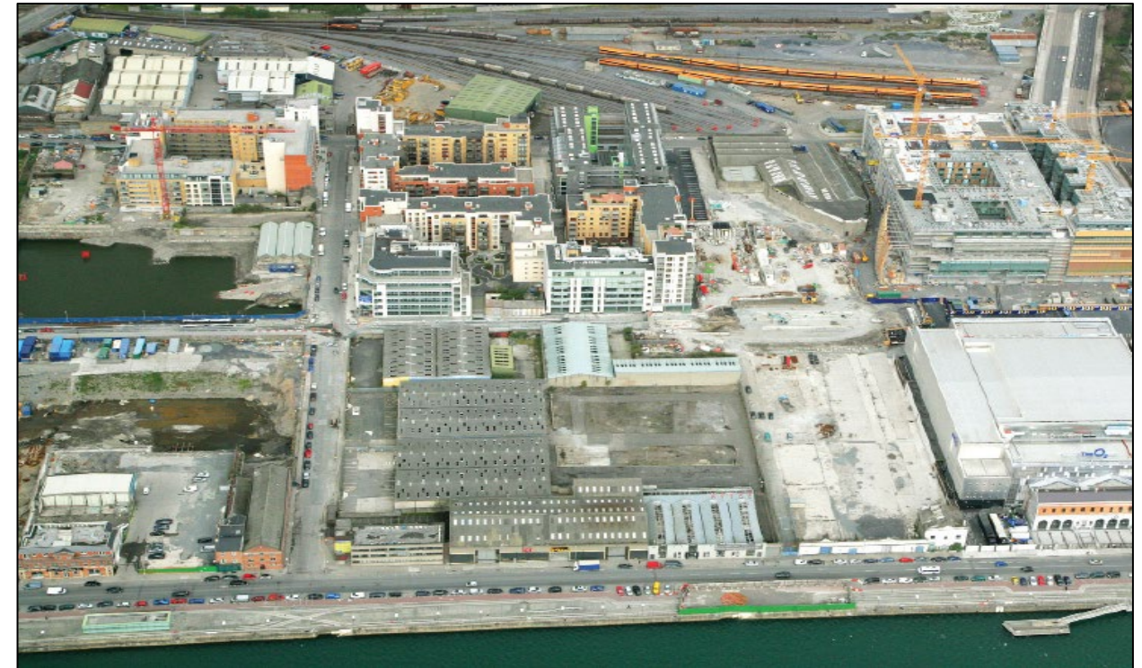
Figure 2.2: Aerial view showing the structure previously located at City Block 9. Source: North Lotts and Grand Canal SDZ Planning Scheme 2014, pg. 195. Cropped by TPA, January, 2021.
