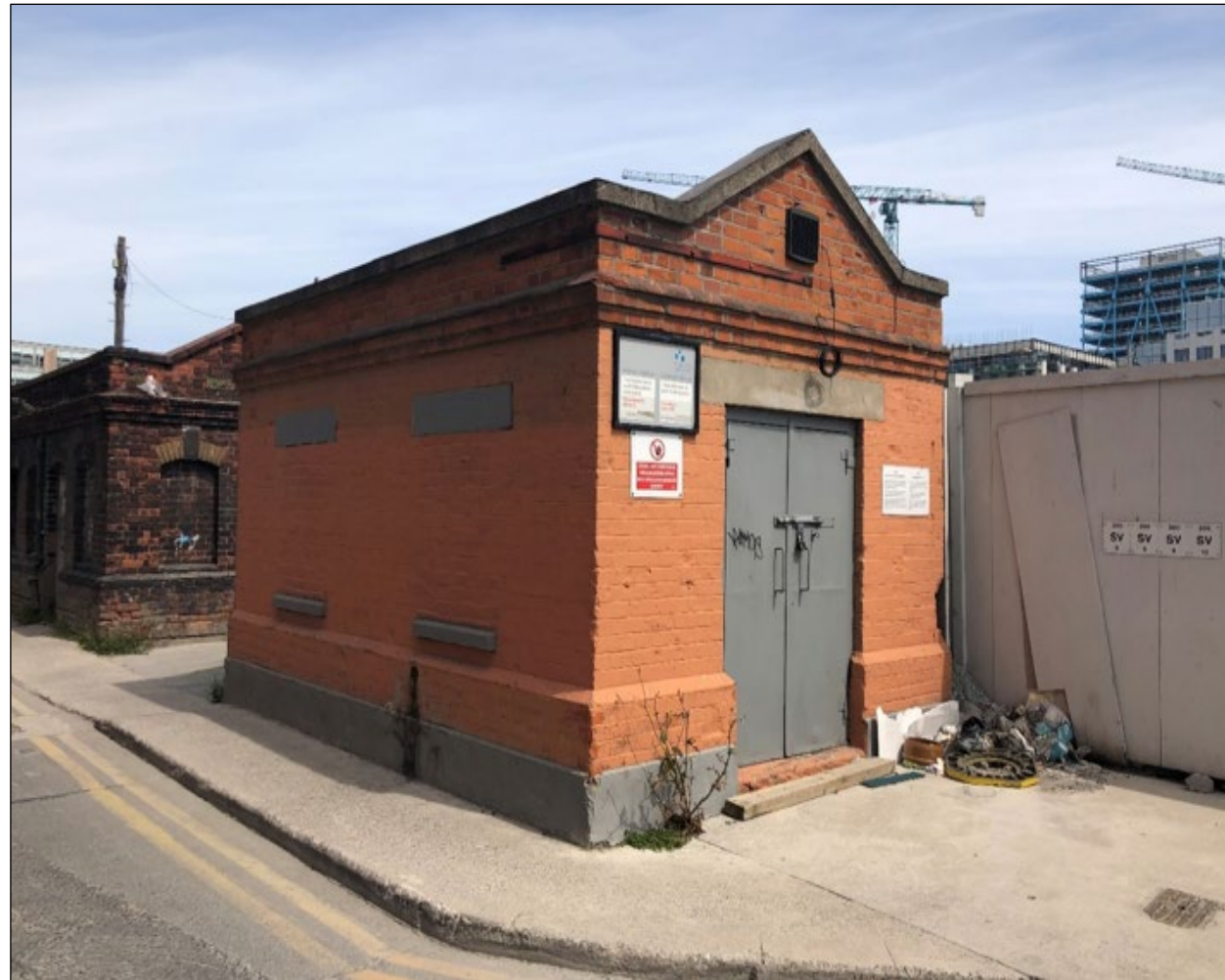
Figure 4.11: Detached single storey electricity substations external to the site on Castleforbes Road. Source: TPA, May 2020.
